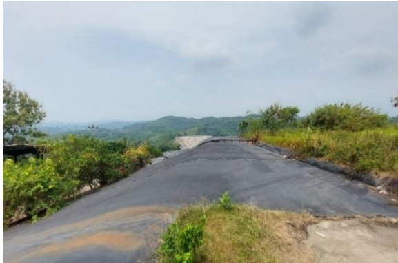
Figure 5. A membrane for a power plant covers waste at the Jatibarang Landfill.
